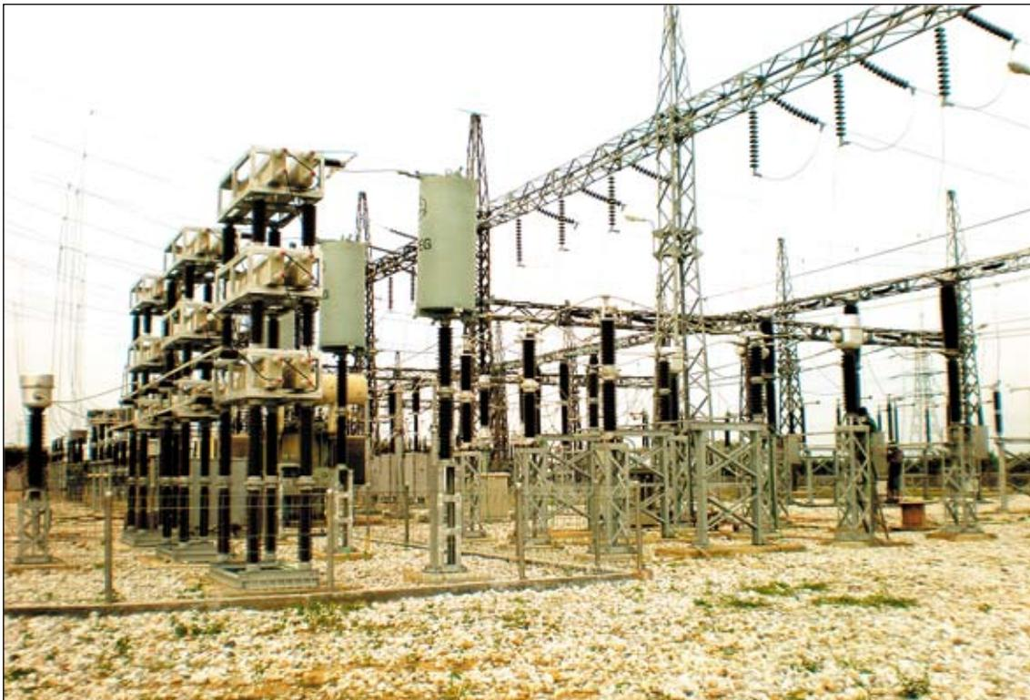
《Capacitor Bank 150kV 25Mvar – GI Duri substation in Indonesia》
